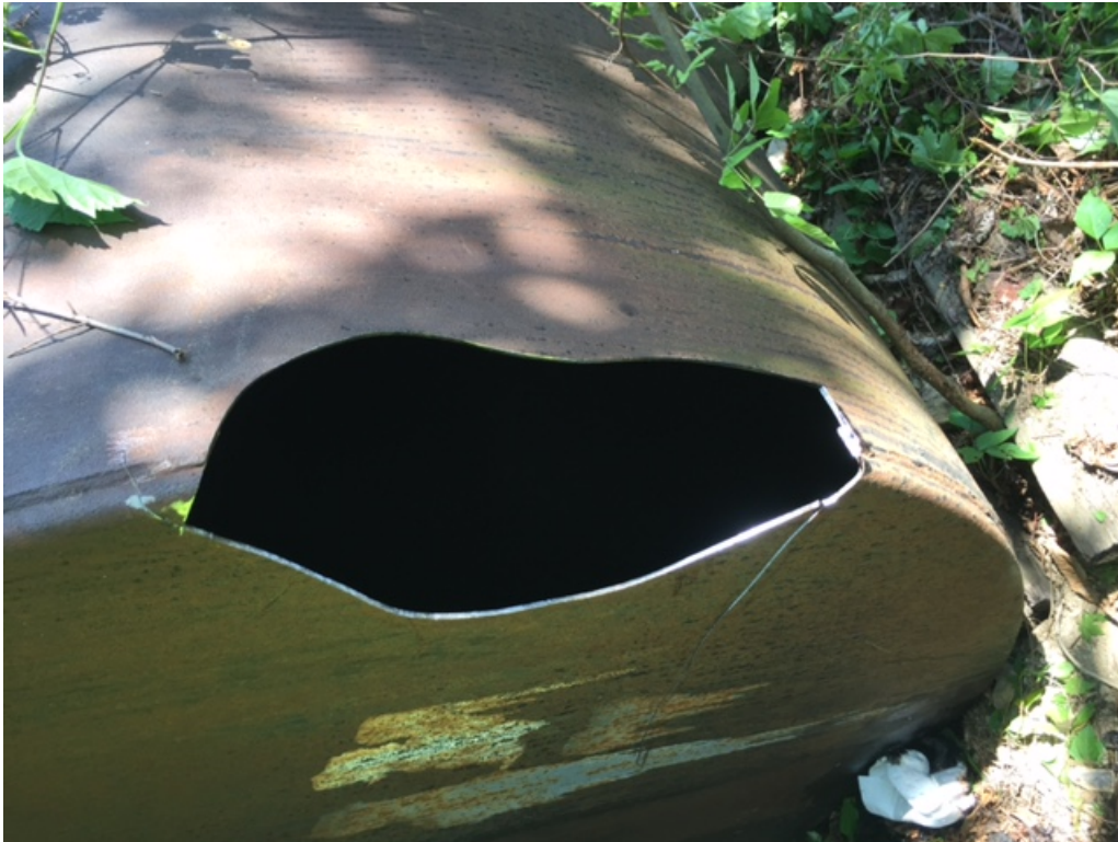
A Large Opening on Tank Side for Interior Cleaning
