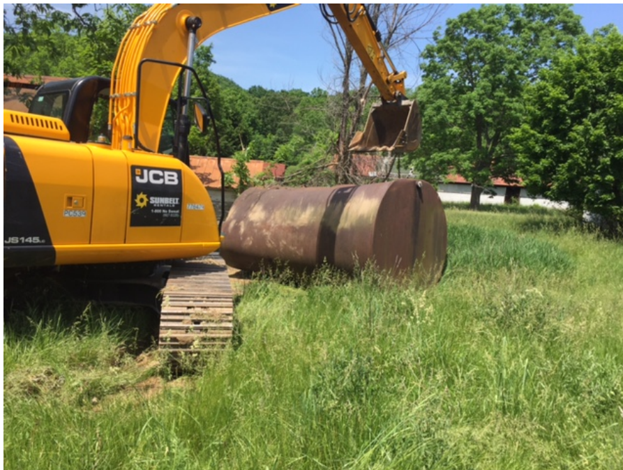
Tank After Cleaning and Removal
