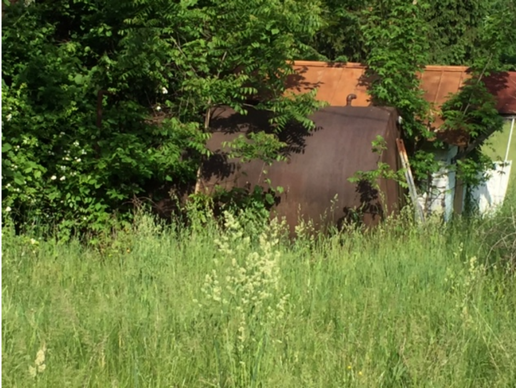
One 4,900-gallon #2 Fuel Oil Aboveground Tank
