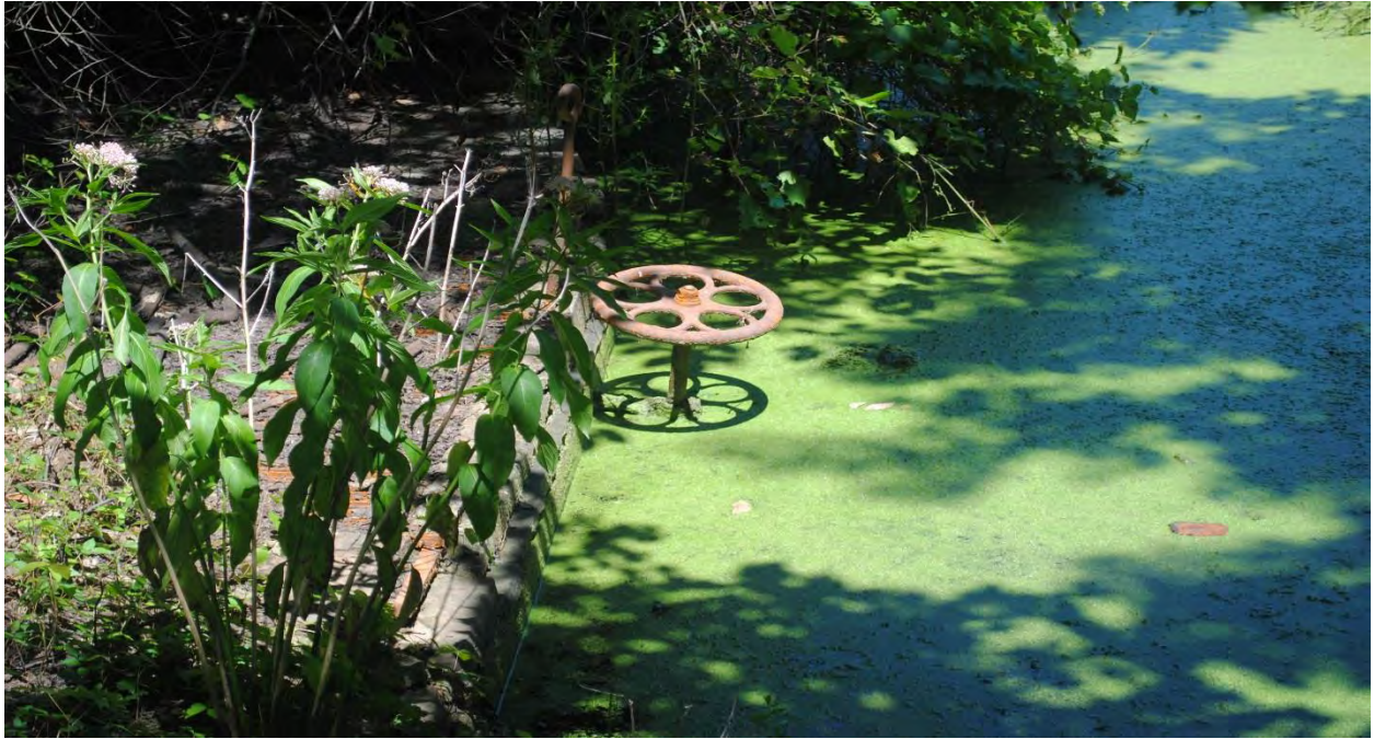
Photo 53: View of the dam located at the southern tip of the wetland. This dam is located 500' north of the M.H. Howell complex and is outside of the APE. Based on the cement and metal hardware, this feature was probably constructed during the late 19 th century to early 20 th century.
