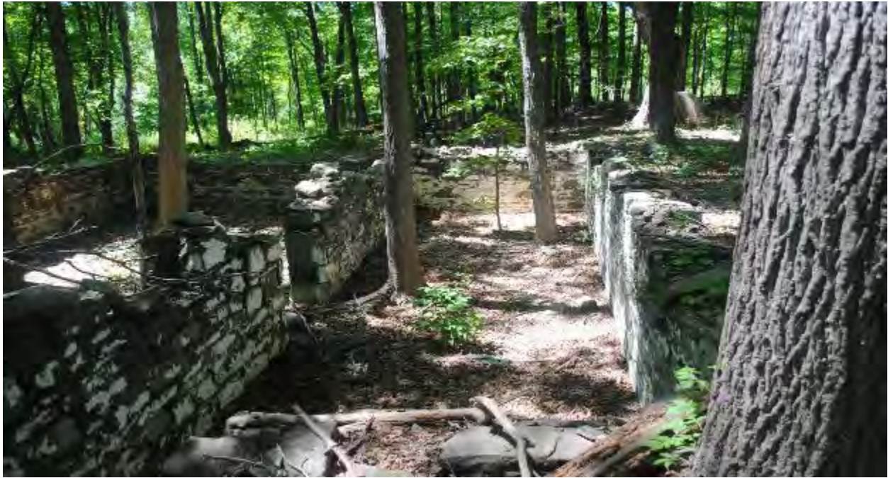
Photo 35: View of a large structure located within the M. H. Howell complex. View to the north.
