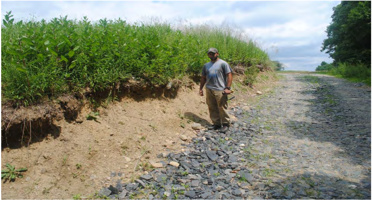
Photo 43: A series of access roads are located throughout the Clovewood Site. View to the north from the southern tier of the Golf Course.
