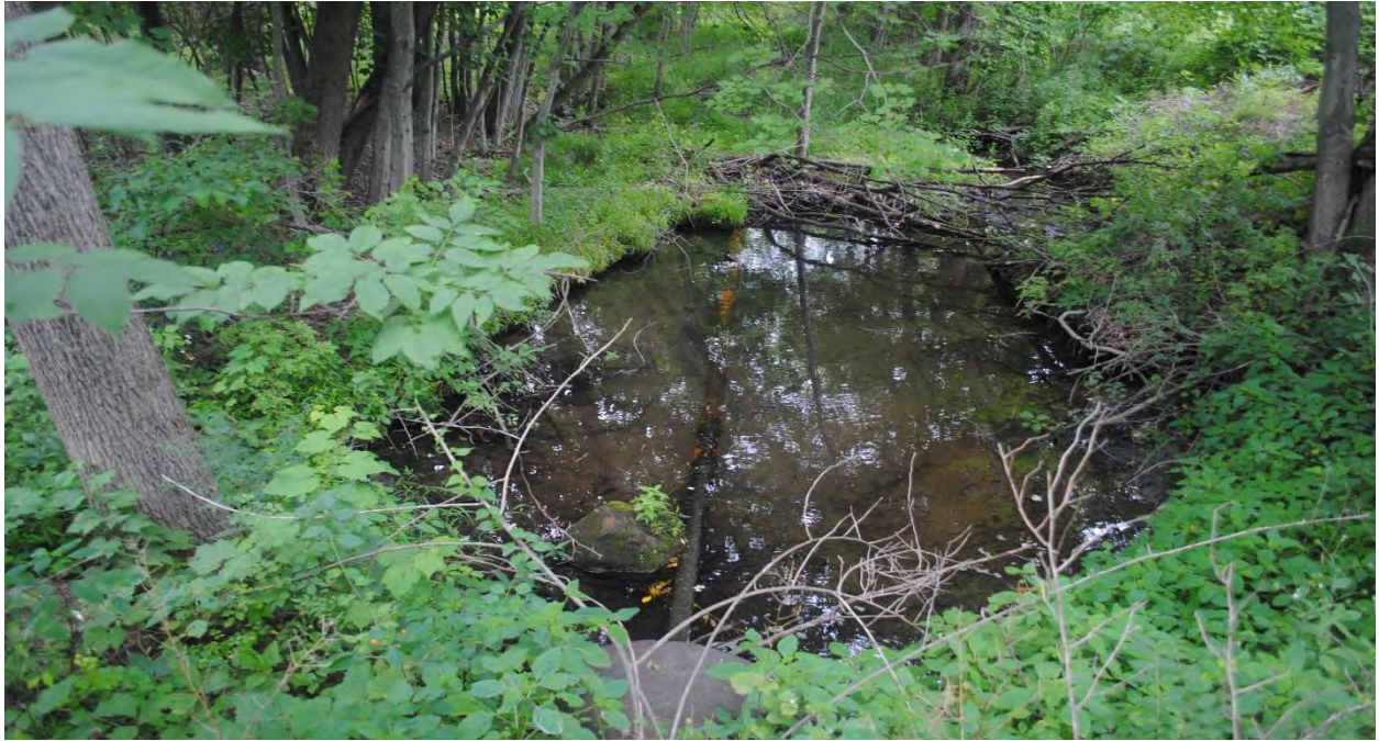
Photo 51: Areas of standing water are located in drainage ditch. View of standing water in Area F.
