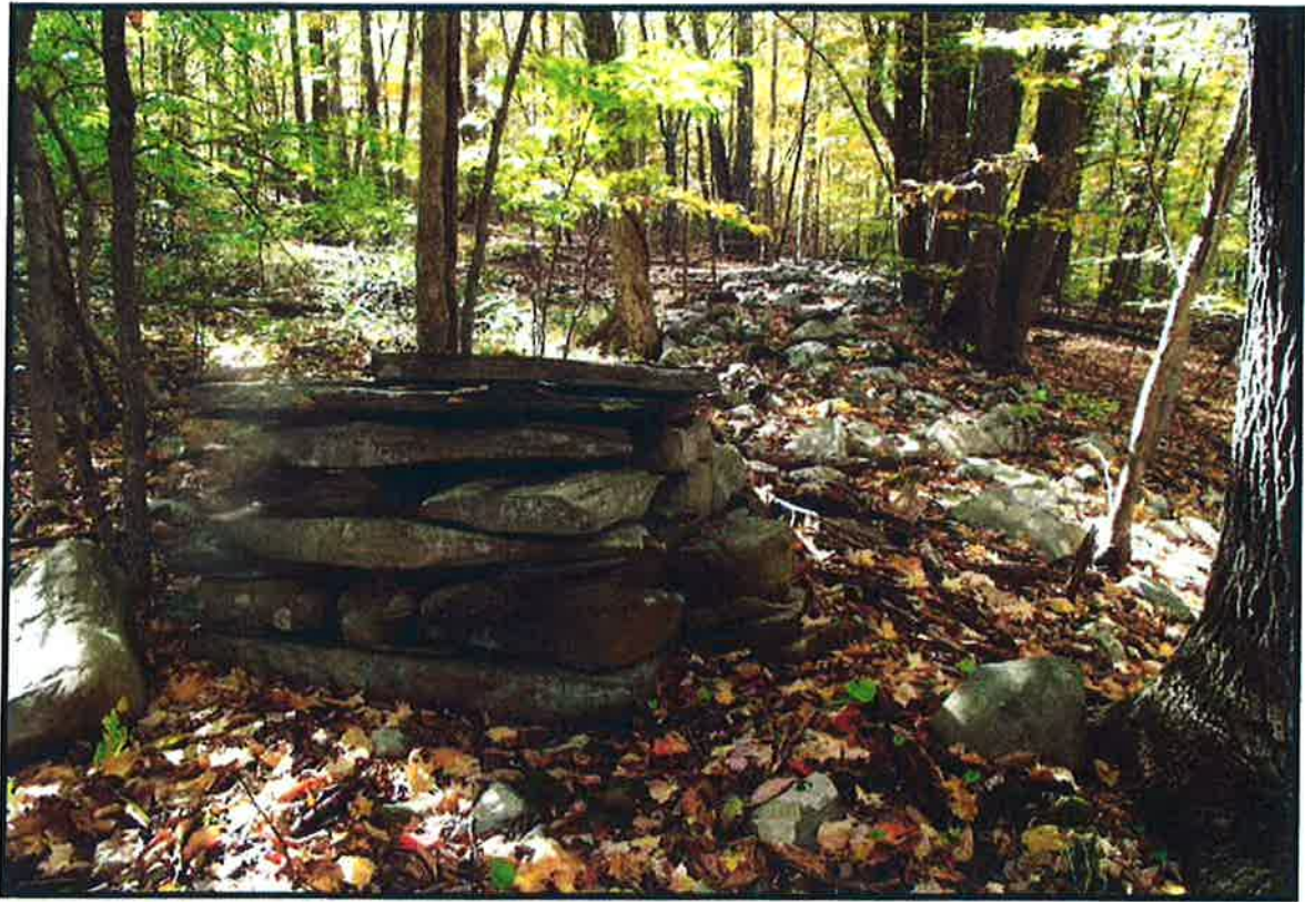
Photograph 23) View of another very typical stone wall on the property.
