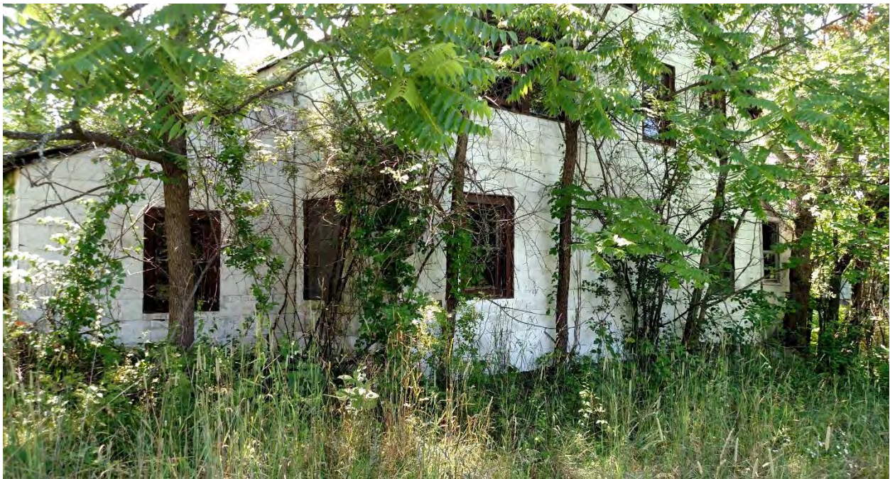
Photo 29: View south of the northern elevation of the H. Howell House.
