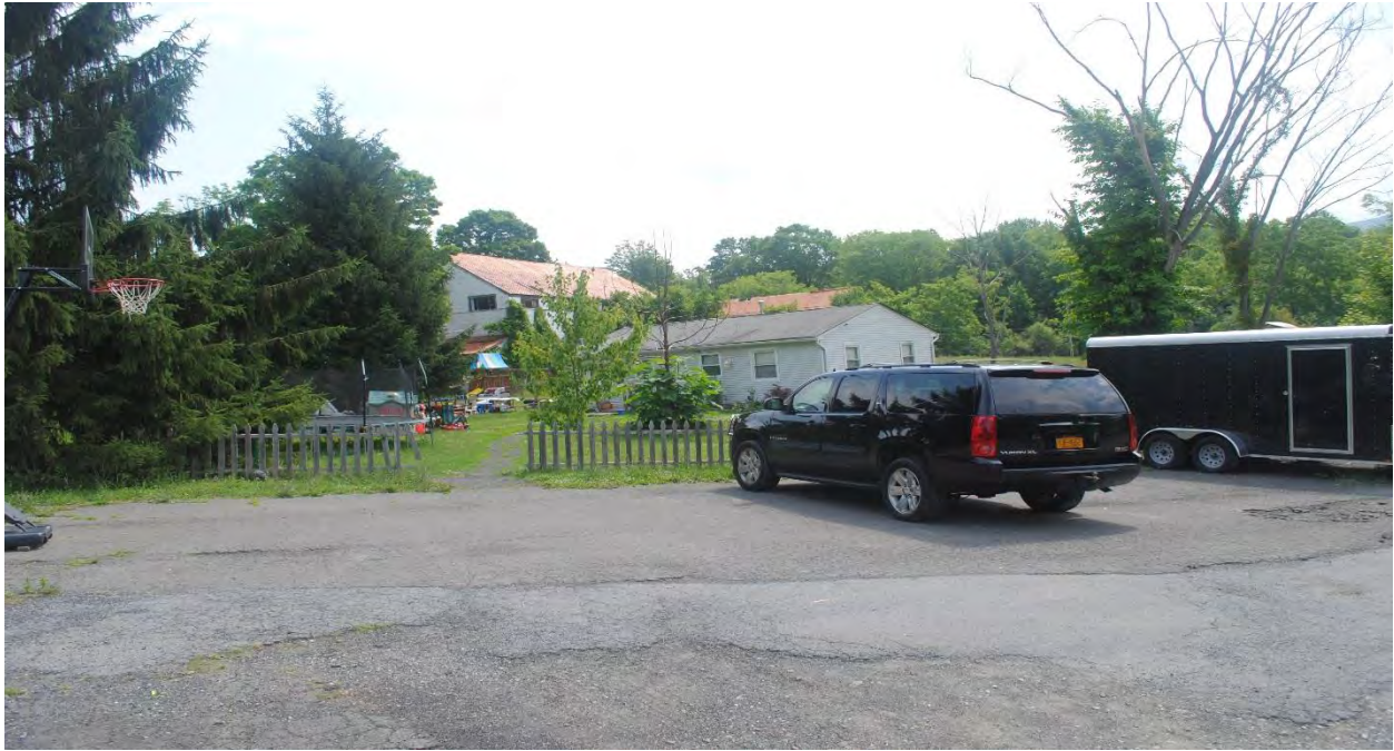
Photo 1: Existing structure located adjacent to the western entry way to the project area. View to the north.
